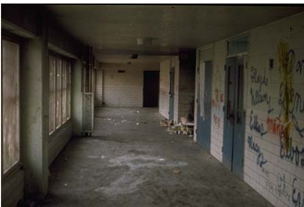
Photo 5: corridor in the final stage.
